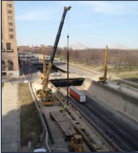
H-pile installation
