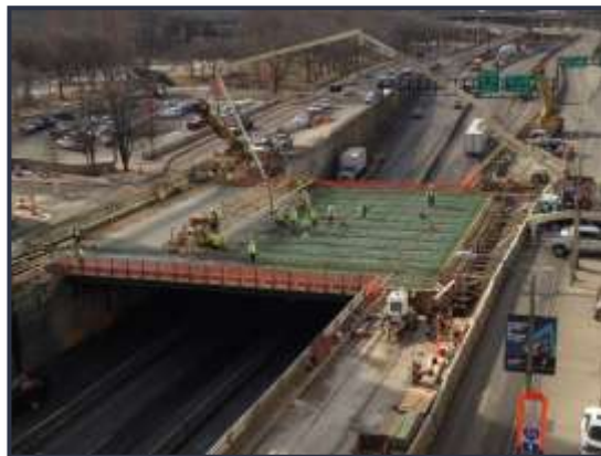
Walnut Street deck placement
