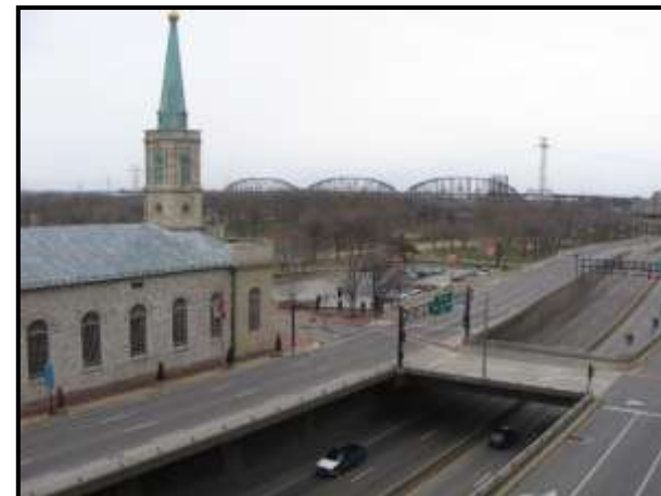
Walnut St. Bridge
